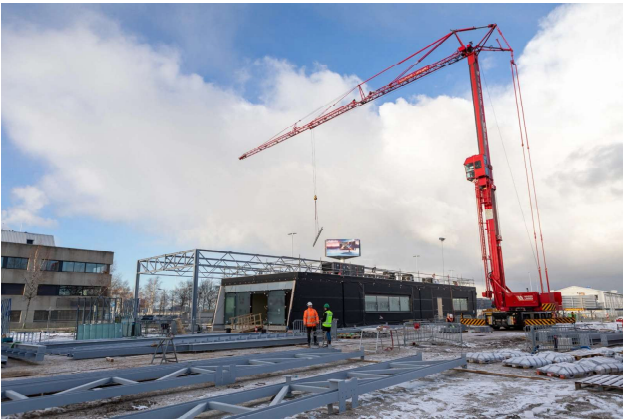
In 2024, we started with the construction of our almost fully circular security checkpoint, Doorlaatpost 90, which we are building by placing existing structures in new positions and using materials from other demolished buildings.
